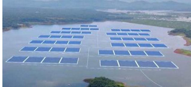
FIGURE 7. Cirata Reservoir Floating Solar Power Plants
